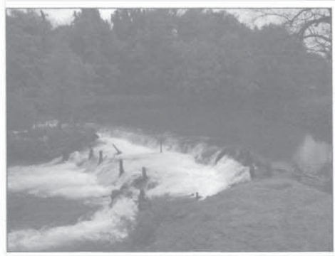
CAPE DAM, ~ 600 CFS, VIEW ACROSS DAM FROM MILLRACE INLET
