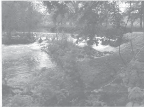
CAPE DAM, ~ 600 CFS, VIEW DOWNSTREAM TO UPSTREAM
