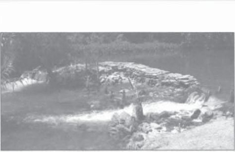
CAPE DAM, ~ 300 CFS, VIEW ACROSS DAM FROM MILLRACE INLET
