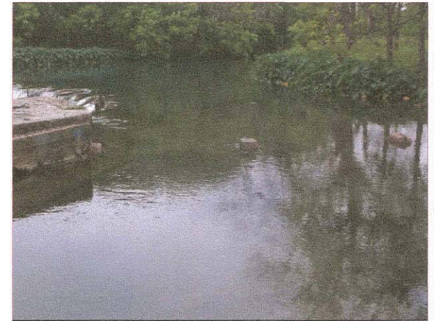
MILLRACE INLET, VIEW DOWNSTREAM TO UPSTREAM The pediments of what once was the Mill Race headgate only begin to be visible when water discharge falls below approx. 280 cfs.
