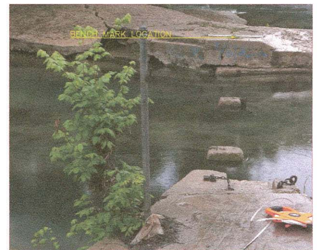
MILLRACE ENTRANCE, VIEW LEFT BANK TO RIGHT BANK
