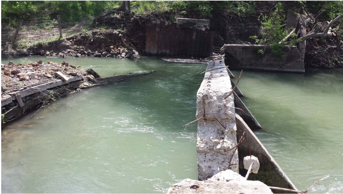
The Ottine Dam Removal Project continues to face delays and setbacks.
